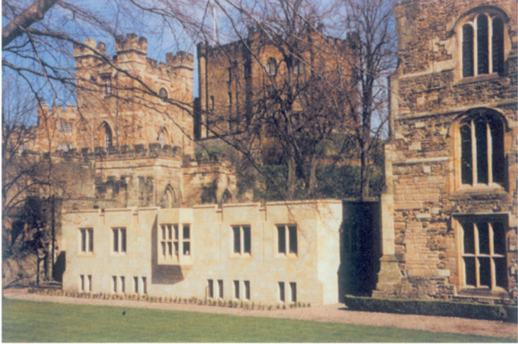
Stonework old and new
